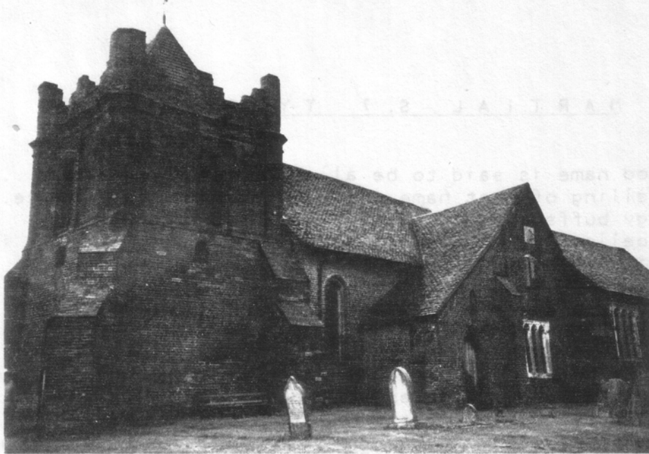
View of the South Side of All Saints Church, East Horndon
